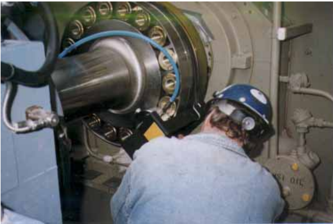
Photo 4 View of 1 1/8 puller tool and safety cage mounted on turbine to coupling flange of 6FA machine. Tool is pressurized and millwright is tightening nut
