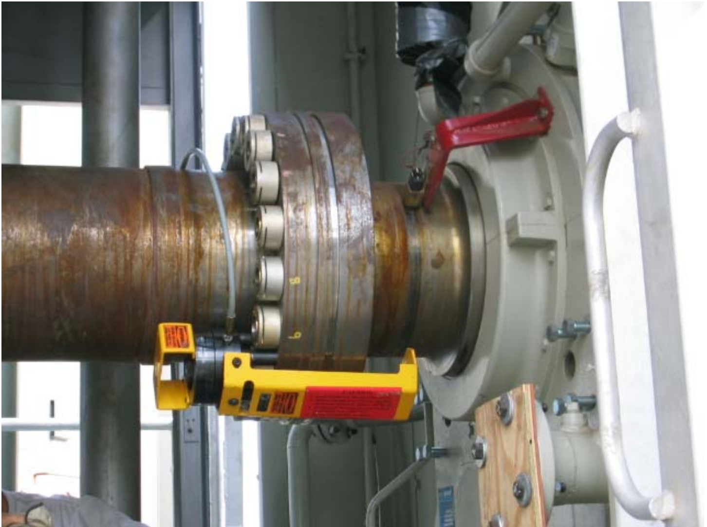
Photo 1 HT-0716 Installed on the Generator End of a 7EA
